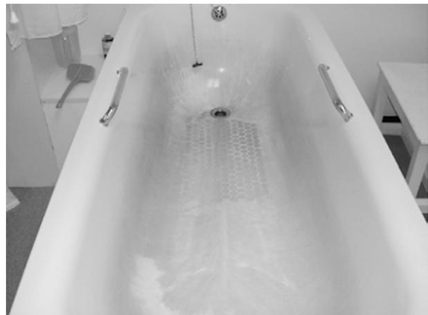
Figure 4. Staining as a result of Silver / Copper ionisation
